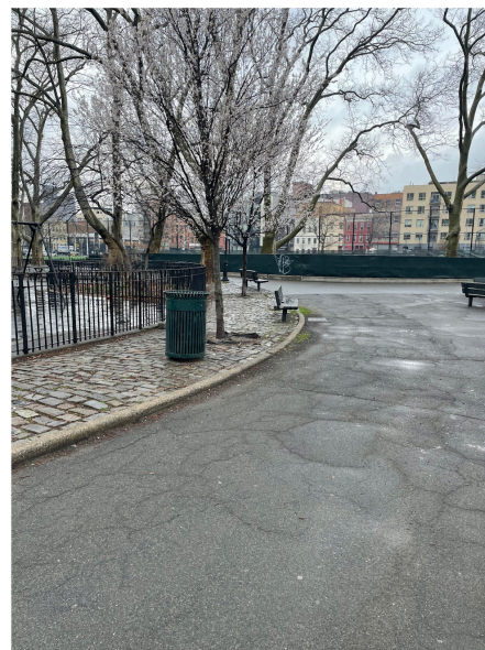
Impermeable surfaces make up a large portion of Sternberg Park
